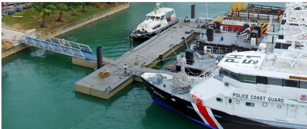
Figure 71: Dock flottant de base 55
